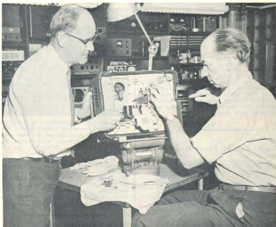
In Projector Maintenance and Repair Shop, Matt Keehan (left), is the 'Sound Man' and Norman Kessel is the 'Picture Man'. Together the two men maintain and repair some 24 projectors throughout the Center, they also maintain the Moviolas at the Center and make necessary repairs for the Marine Corps in the Metropolitan area. They design projection equipment for special usage and put on Projection shows for all requesting government agencies. Both men have been on the job for more than 19 years each.
